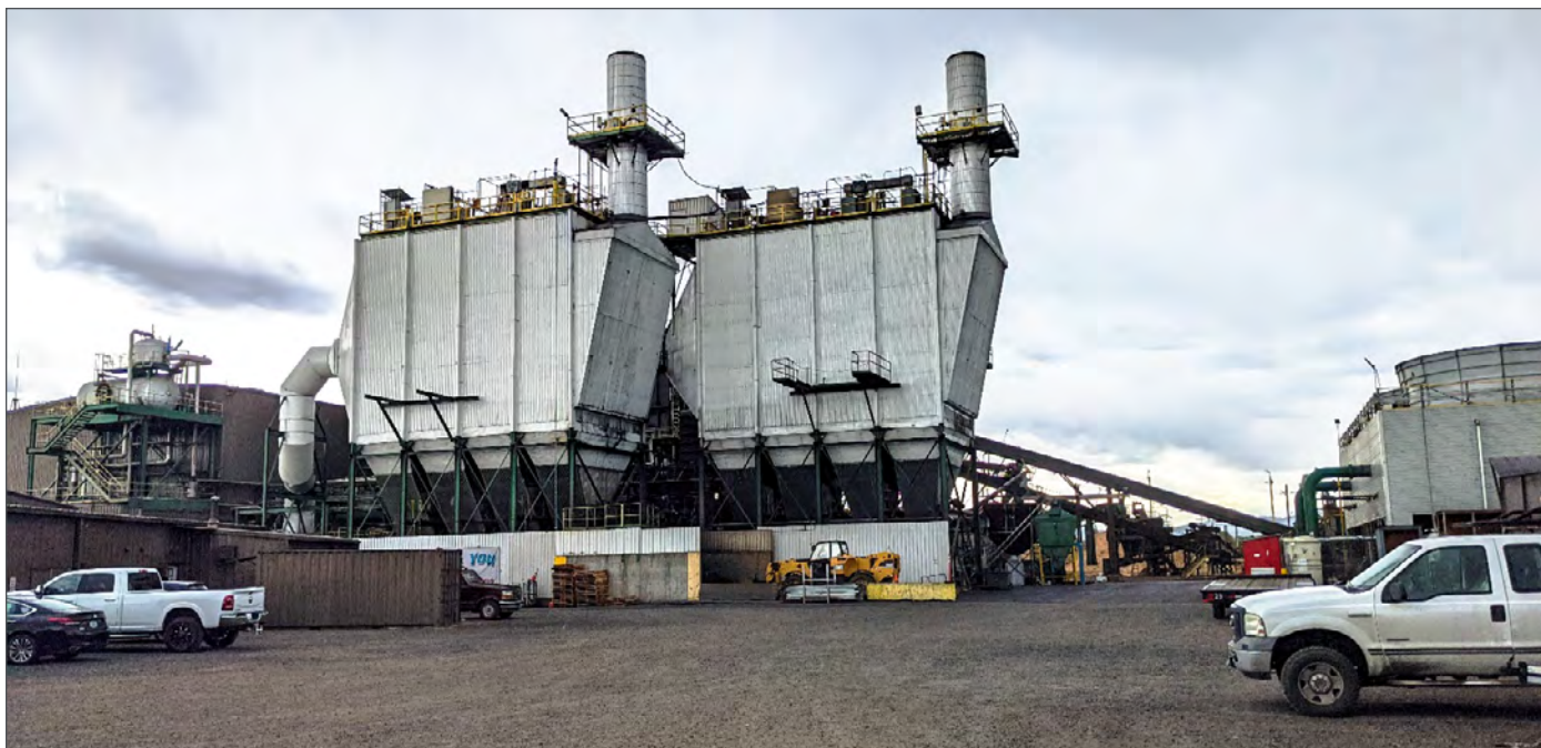
Figure 1.3. Biomass One in Medford, Oregon is a biomass power plant generating 32.5 megawatt electrical (MWe) (28.5 MWe goes to the grid). This plant consumes 200,000 tons per year of dry biomass and can recover 50,000 cubic yards of biochar annually (Photo: Karl Strahl)
