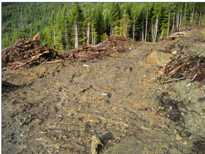
Figure 5.6. This forest road is to be permanently deactivated after completion of timber harvest operations near Humboldt, California. (Photo: Han-Sup Han)
